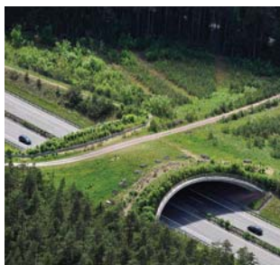
a Highway overpass
