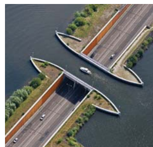
c Canal overpass
