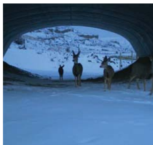
b Highway underpass
