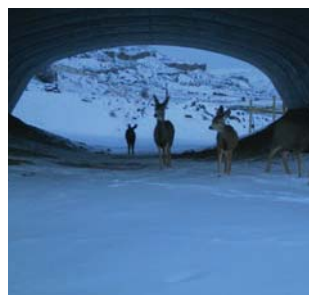
b Highway underpass
