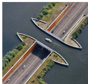
c Canal overpass
