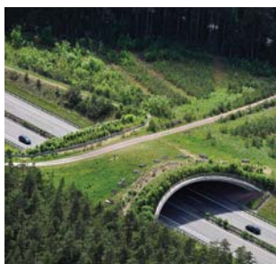
a Highway overpass
